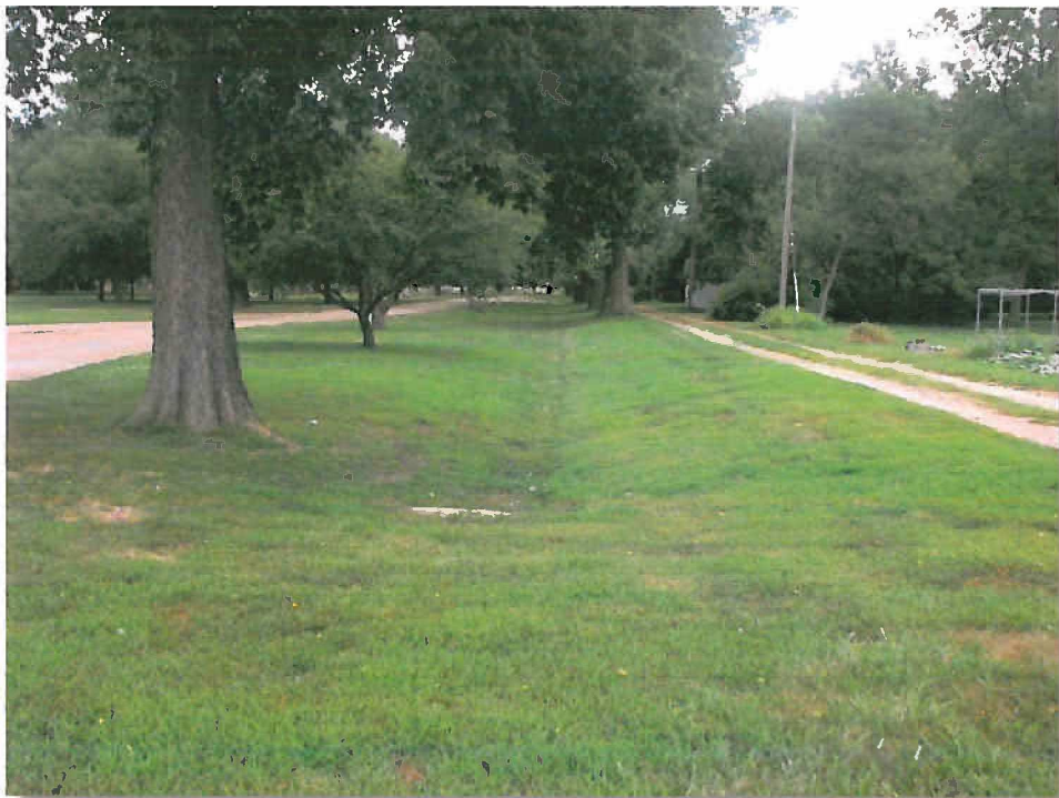
Photo 5.8 View looking east at south end of city park near the RV dumping station. Drainage swale collects runoff from the east and enters inlet as shown.
