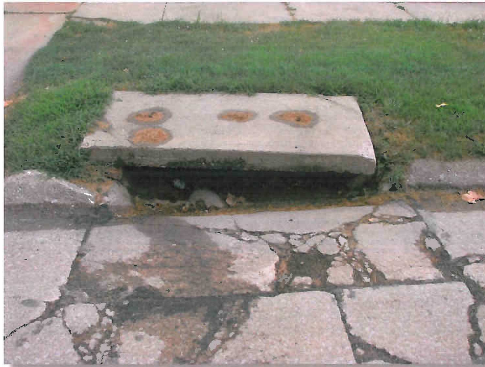
Photo 5.5 View looking south at the city park entrance on W. 8 th Street and Maple Street. Two existing inlets on Maple Street completely filled with debris.
