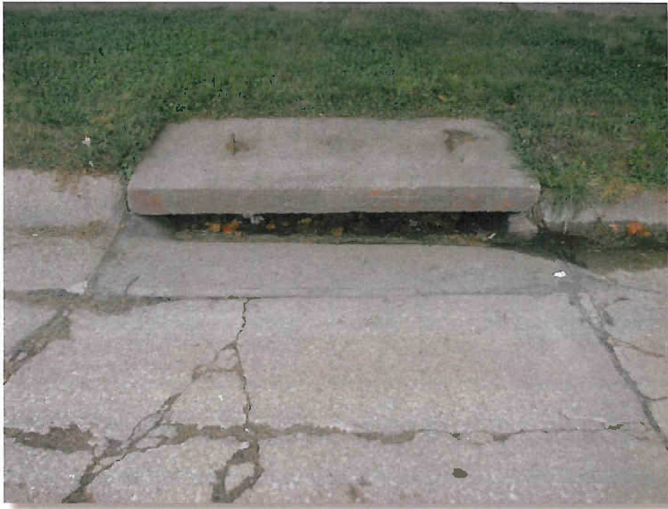
Photo 5.7 View of inlet on west side just north of W. 8 th and Maple Street. Debris has collected in the inlet. Inlet connects to storm sewer system on west side of City Park.
