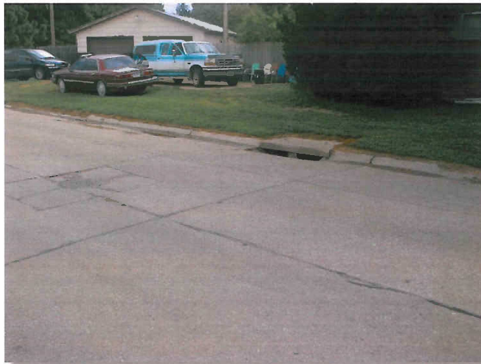
Photo 5.12 View looking north on Fredrick Street just north of W. 4 th Street. Existing curb inlet on the east side collects runoff into the system which discharges into the Little Blue River.
