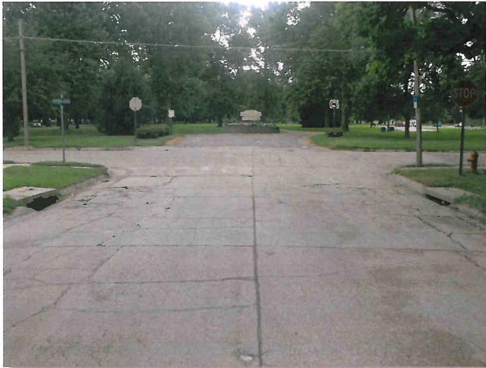
Photo 5.5 View looking south at the city park entrance on W. 8 th Street and Maple Street. Two existing inlets on Maple Street completely filled with debris.
