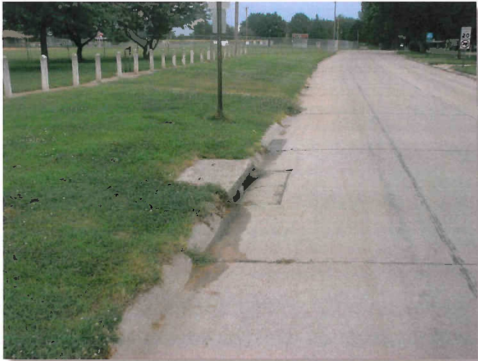
Photo 5.11 View looking north on Fredrick Street just north of W. 4 th Street. Existing curb inlet on the west side collects runoff into the system which discharges into the Little Blue River.
