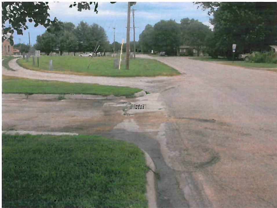
Photo 5.14 View looking north on Fredrick Street on the west side at entrance drive of maintenance building. Inlet appeared to be free of debris. Connects to storm sewer which discharges into the Little Blue.
