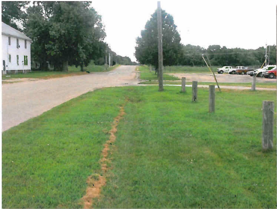
Photo 5.13 View looking south on Fredrick Street on the west side. Drainage ditch and existing inlet shown toward the drive. Inlet covered in grass.
