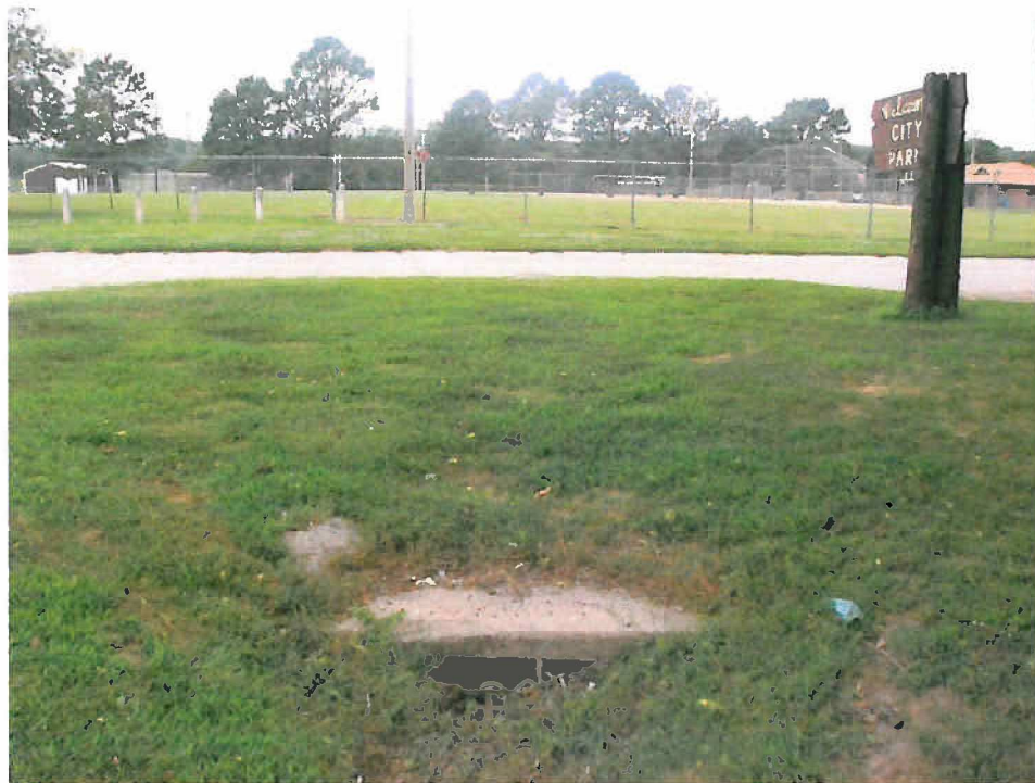
Photo 5.9 View looking west at inlet by the RV dumping station on the southwest side of the city park. Inlet collects runoff and ties into the storm sewer system on the west side of Fredrick Street.
