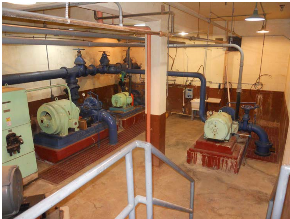
Figure IV-6: High Service or Booster Pumps from the Underground Reservoir
