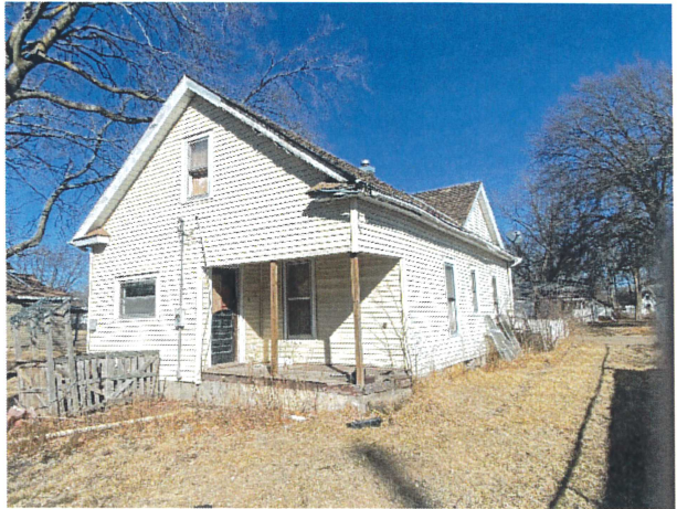
Southeast exterior elevation viewing northwest
