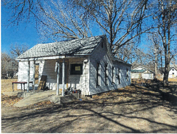
Southeast exterior elevation viewing northwest
