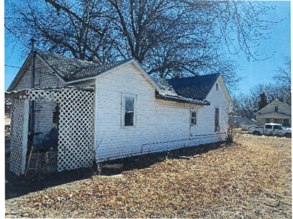
Northwest exterior elevation viewing southeast
