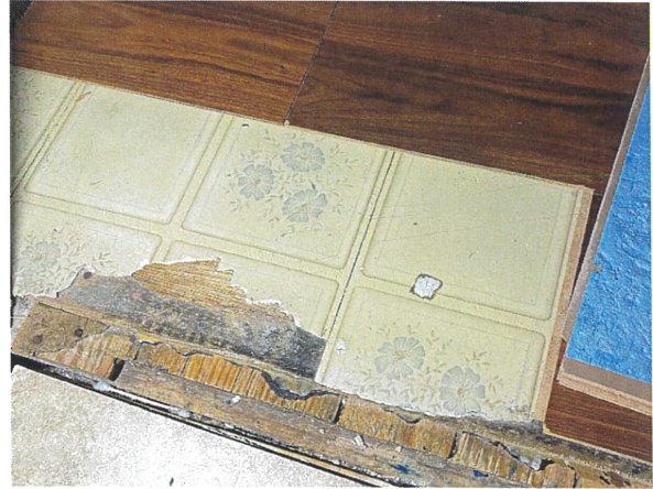
FAI-204-100223-001, 002, 003 None Detected, Cream Vinyl Sheet Flooring
