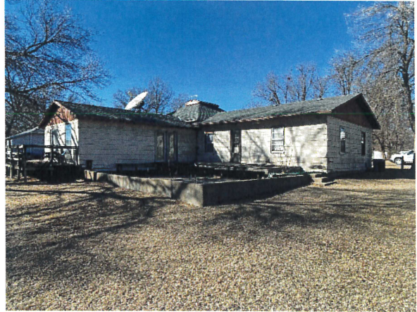
Southeast exterior elevation viewing Northwest
