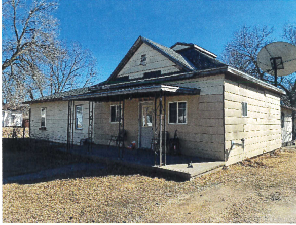
Northwest exterior elevation viewing southeast
