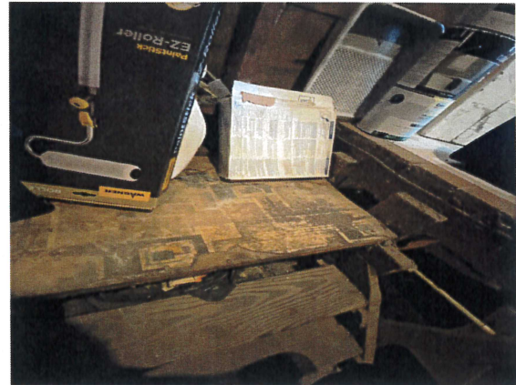
FAI-306-090223-025, 026, 027 None Detected, Multi-colored Vinyl Sheet Flooring
