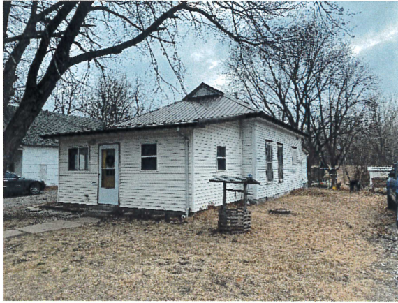
Northwest exterior elevation viewing southeast
