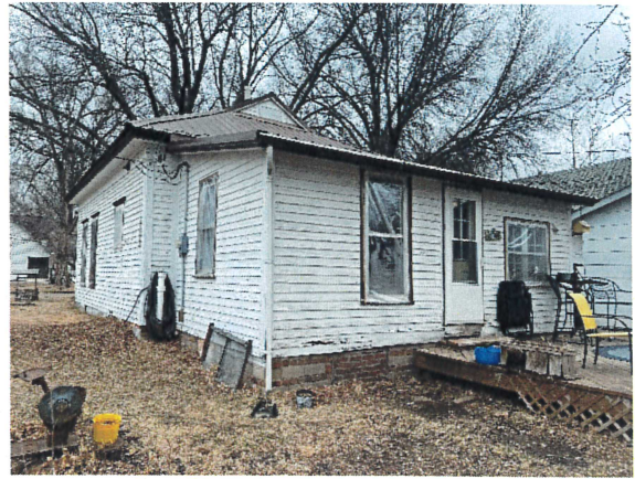
Southwest exterior elevation viewing Northeast
