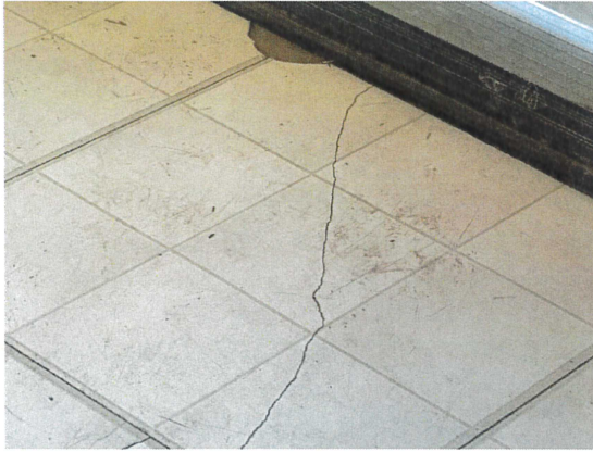
FAI-306-090223-001, 002, 003 None Detected, 12" x 12" White Vinyl Floor Tile
