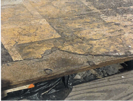
FAI-306-090223-025, 026, 027 None Detected, Multi-colored Vinyl Sheet Flooring
