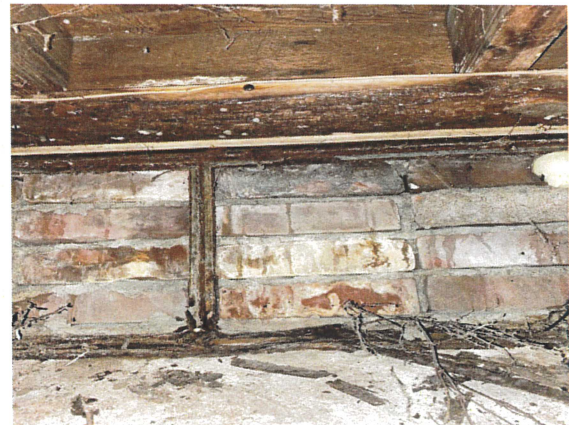
FAI-306-090223-028, 029, 030 None Detected, Gray Window Glazing
