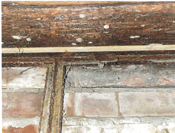
FAI-306-090223-028, 029, 030 None Detected, Gray Window Glazing
