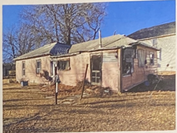
Northeast exterior elevation viewing southwest
