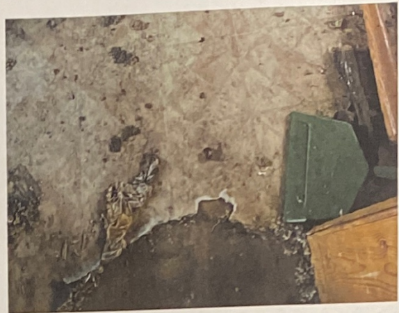
FAI-321-130223-001, 002, 003 None Detected, Tan Vinyl Sheet Flooring
