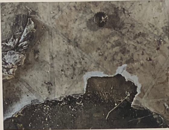
FAI-321-130223-001, 002, 003 None Detected, Tan Vinyl Sheet Flooring
