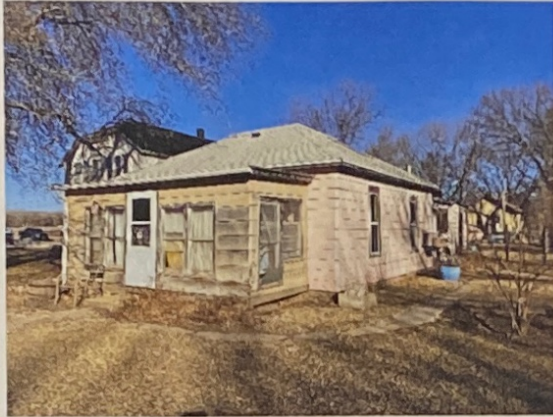
Southeast exterior elevation viewing northwest
